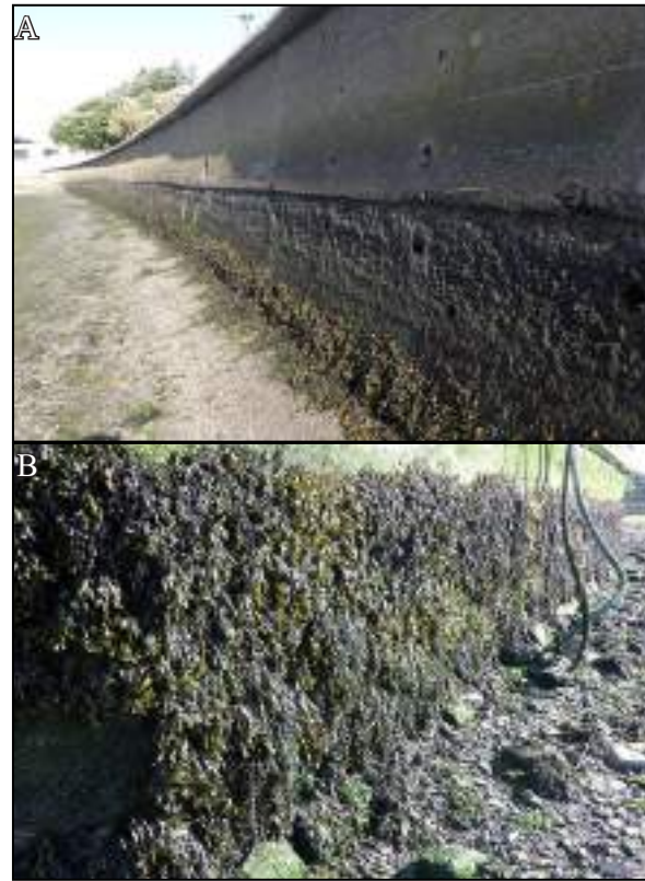
Fig. 504. General habitat: The habitat was consistent throughout the survey, primarily characterized by a concrete wall.
