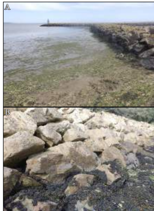
Fig. 495. General habitat: The habitat was consistent throughout the survey, primarily characterized by breakwater stones.
