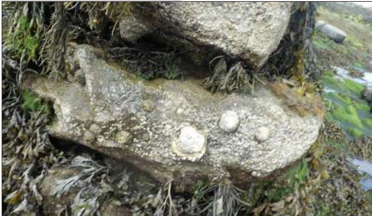
Fig. 232. Pacific oysters on the stone building blocks of the pier.
